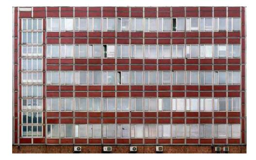
Emalite glass is a synthetic opaque and multicoloured glass that appeared in the 1950s. Inserted in aluminium frames, it is used to cover the facades of buildings with modular panels of any requested colour. Its simplicity of use as well as its modularity account for its popularity in the 60s and 70s in Western Europe and in the countries of the socialist bloc. However, emalite glass does not age well, and is often replaced by other covering material, not as colourful.
